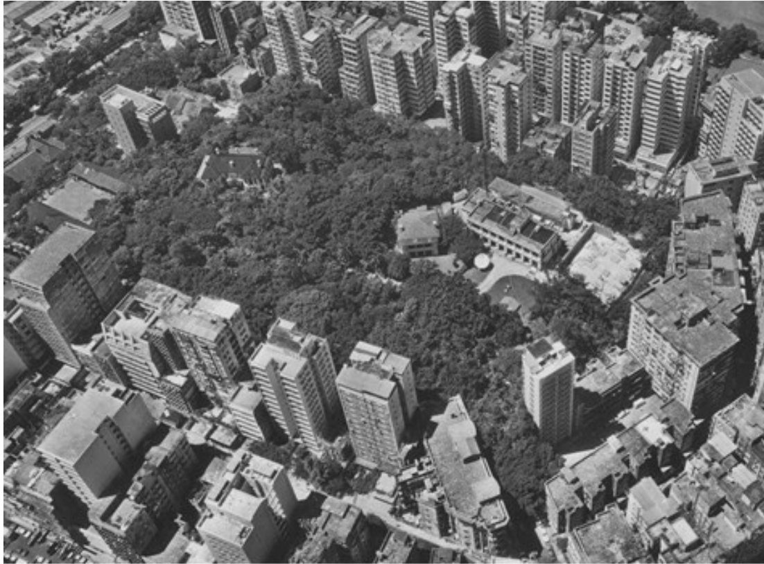
Figure 24. An aerial view of the Observatory in September 1979, with the construction of the Centenary Building to the right of the Main Building (courtesy of Survey and Mapping Office, Lands Department)
