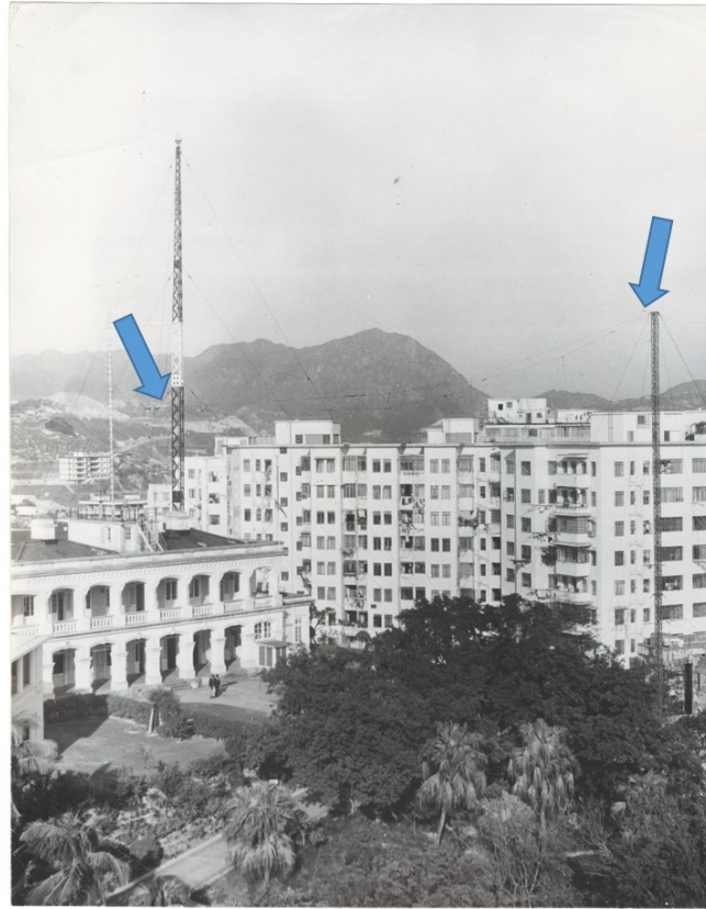
Figure 20. Photo of aerial network around 1969-1970 (Photo courtesy of Mr Shun Chi-ming, Director of the Hong Kong Observatory, 2011-present)
