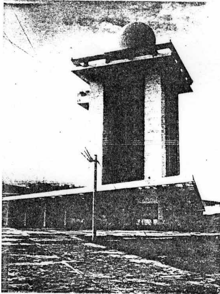
10.5(7) Fig. 10.17 The 30 m tower at Hua Lien on the east coast of Taiwan with a Raytheon WSR 64 M 100 mm weather radar. The dome and radar were blown off the tower in typhoon Gilda 18th November 1967. (Photo by Bocks 1967)
