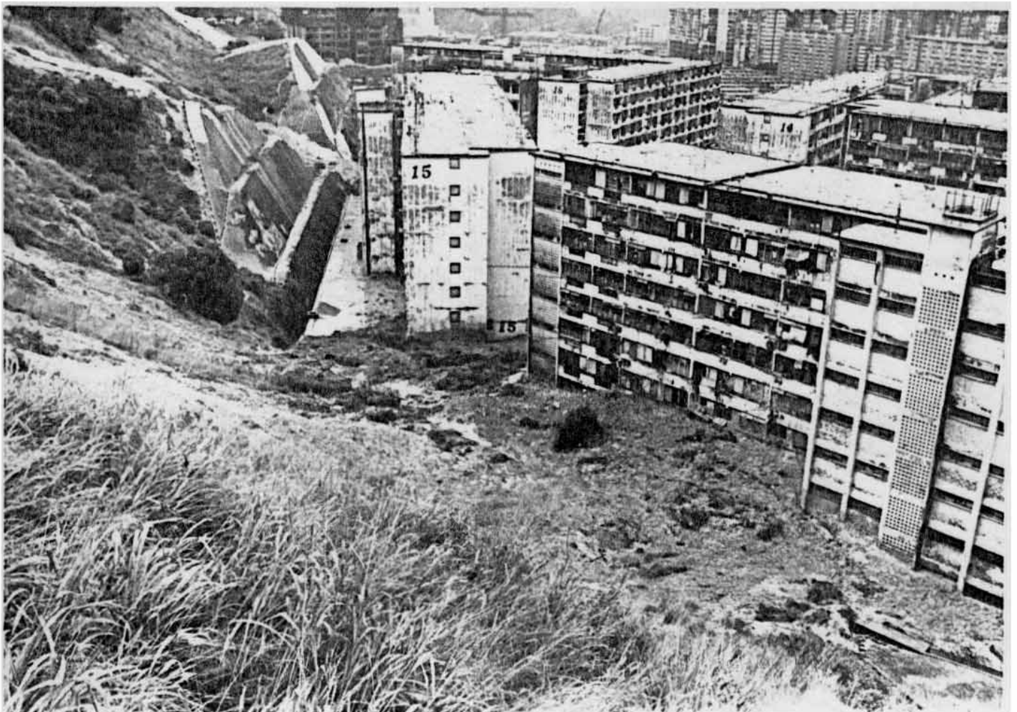
Fig. 6.8.1 5 A mud avalanche in a filled slope at Sau Mau Ping, Hong Kong caused by tropical storm Ellen on 25th August 1976. (Hong Kong Standard.)
