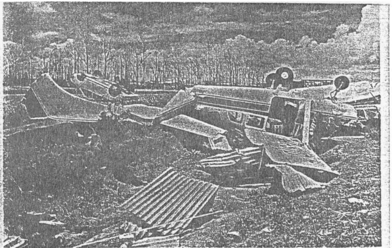
Part of the damage at Darwin Airport.
