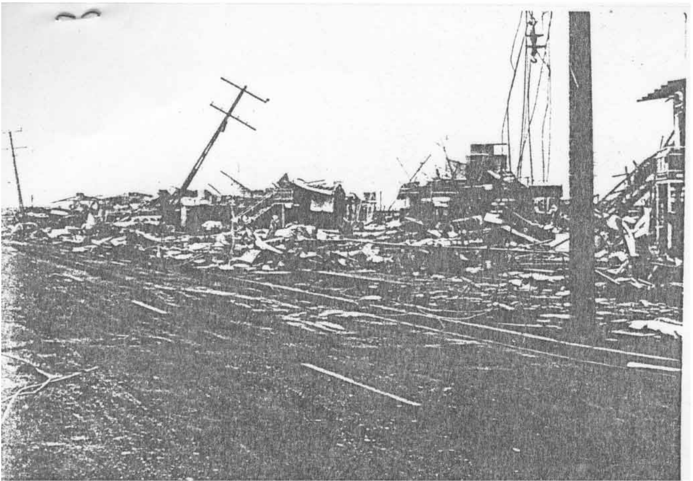
Fig. 5. 1(2) Darwin houses with roof and upper storeys missing. (Photo by Andrew Fraser)
