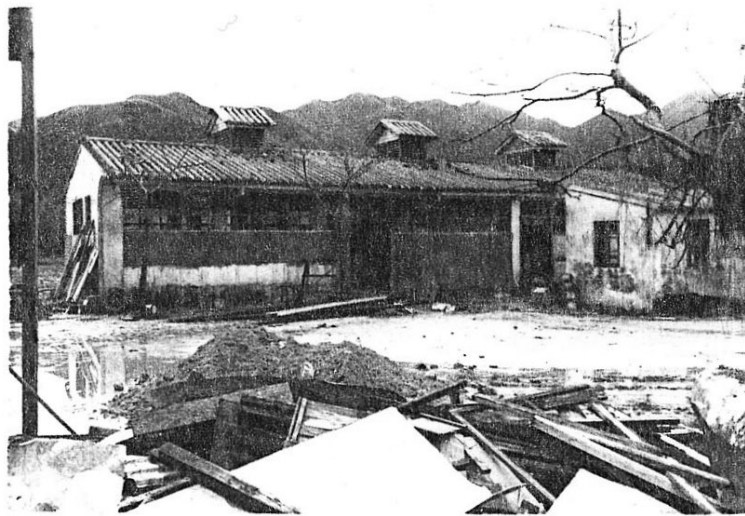
Fig. 5.4 . An old building with roof intact after the passage of typhoon Wanda 1962 at Hong Kong. Retention of the roof was probably due to the equalisation of pressure through the ventilators on the eaves. Note lack of leaves on the trees and debris - either wind or water borne - on the tree at right. (From Peterson and Cheng 1966.)
