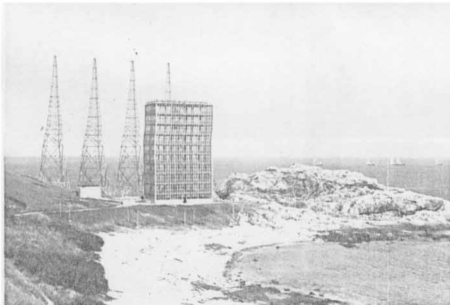
Fig. 5. . The ten-storey building at Cape D'Aguilar, Hong Kong which was built to study wind effects. The four 61 m masts carry 20 anemometers.
