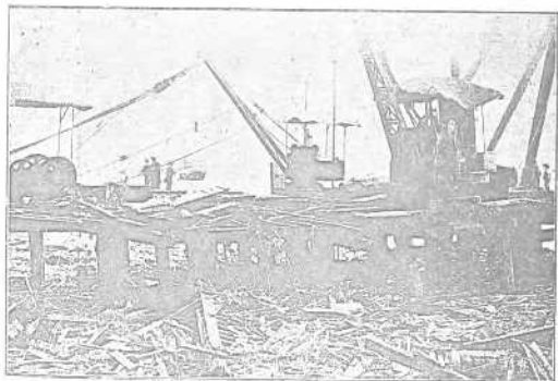
A damaged wharf at Kowloon.
