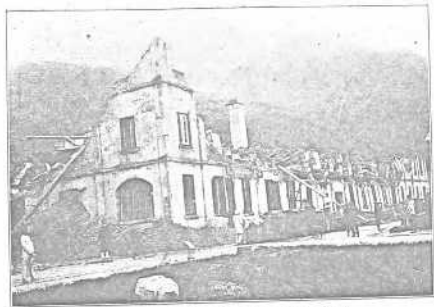
Another view of a damaged godown at West Point
