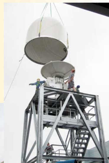
▲ Figure 2: Installation of radome by radar technical personnel.
