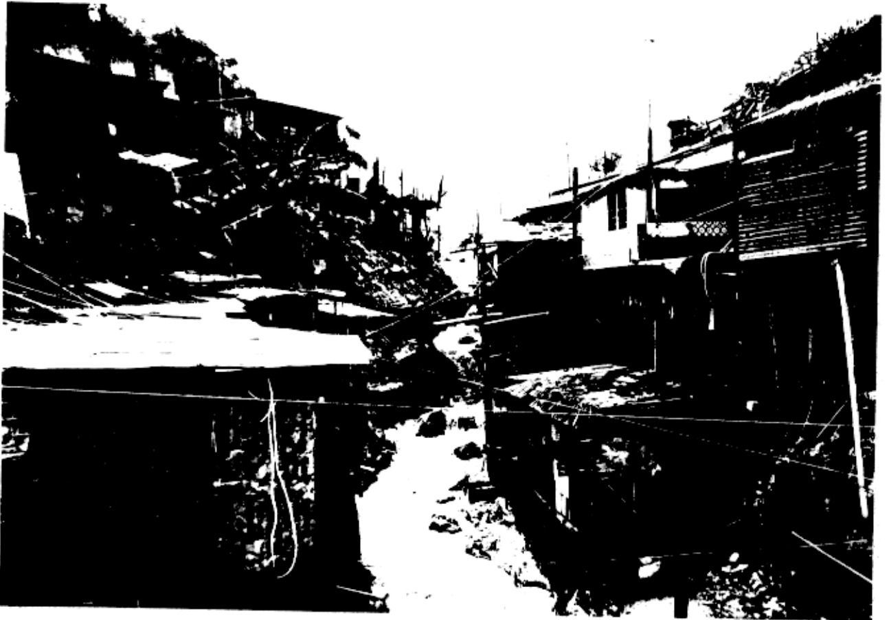
Plate 13. Flooding in the squatter area, Sau Mau Ping
