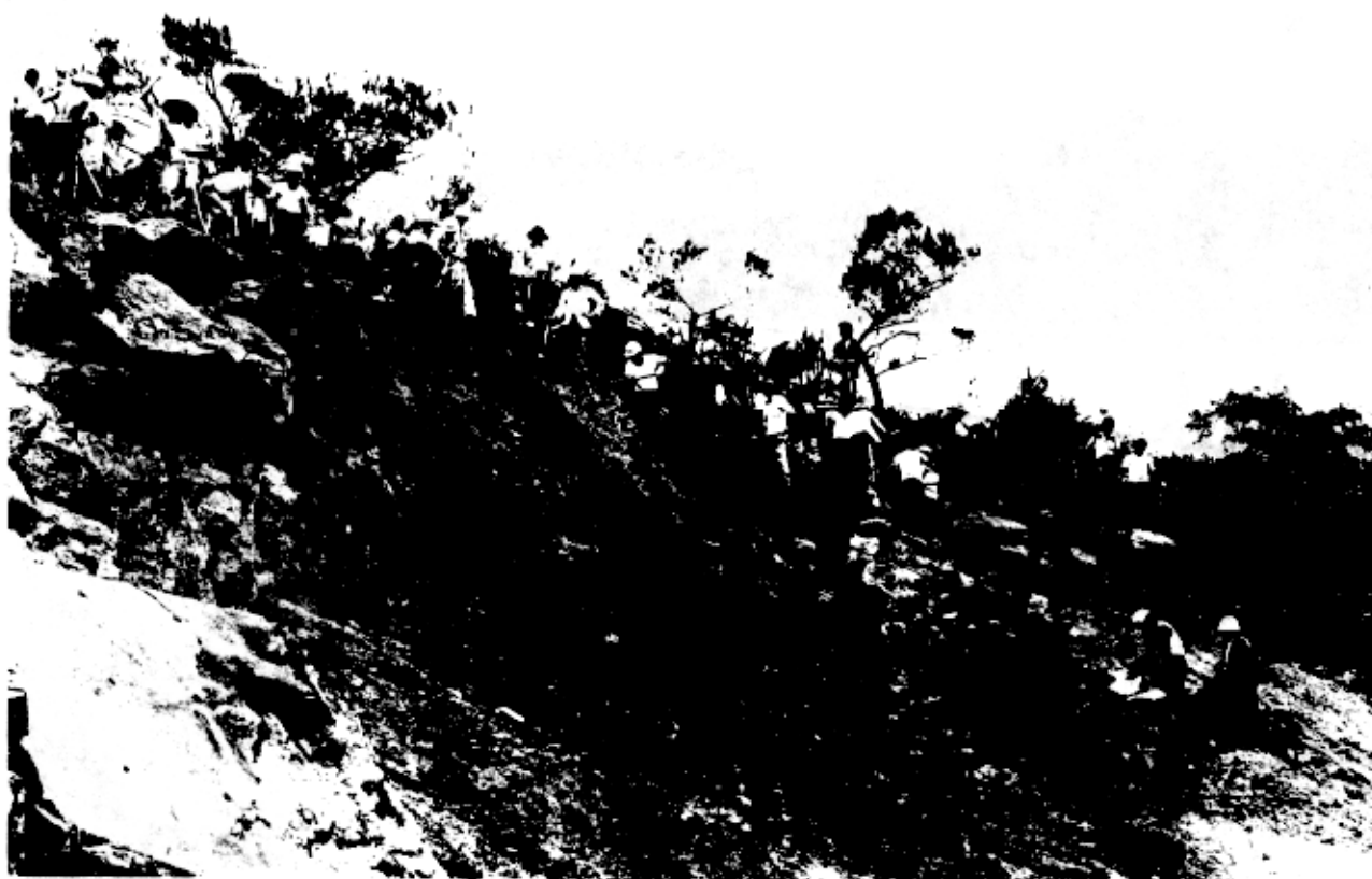
Plate 9. Close-up view of the landslip area on Tuen Mun Road
