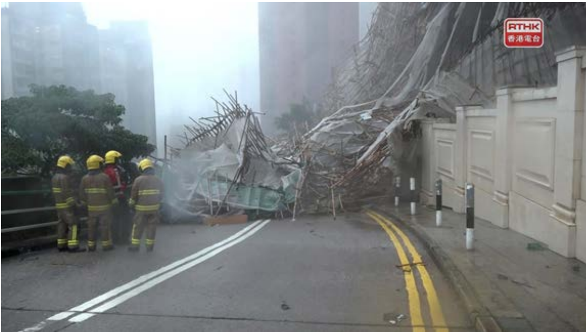
圖 3.5.8a 二零二一年十月八日跑馬地有棚架倒塌。(圖片由香港電台提供) Figure 3.5.8a Scaffolding collapsed in Happy Valley on 8 October 2021. (Courtesy of Radio Television Hong Kong)
