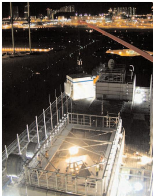
Figure 4 — Lifting the LIDAR onto the roof-top of the Air Traffic Control complex at HKIA
