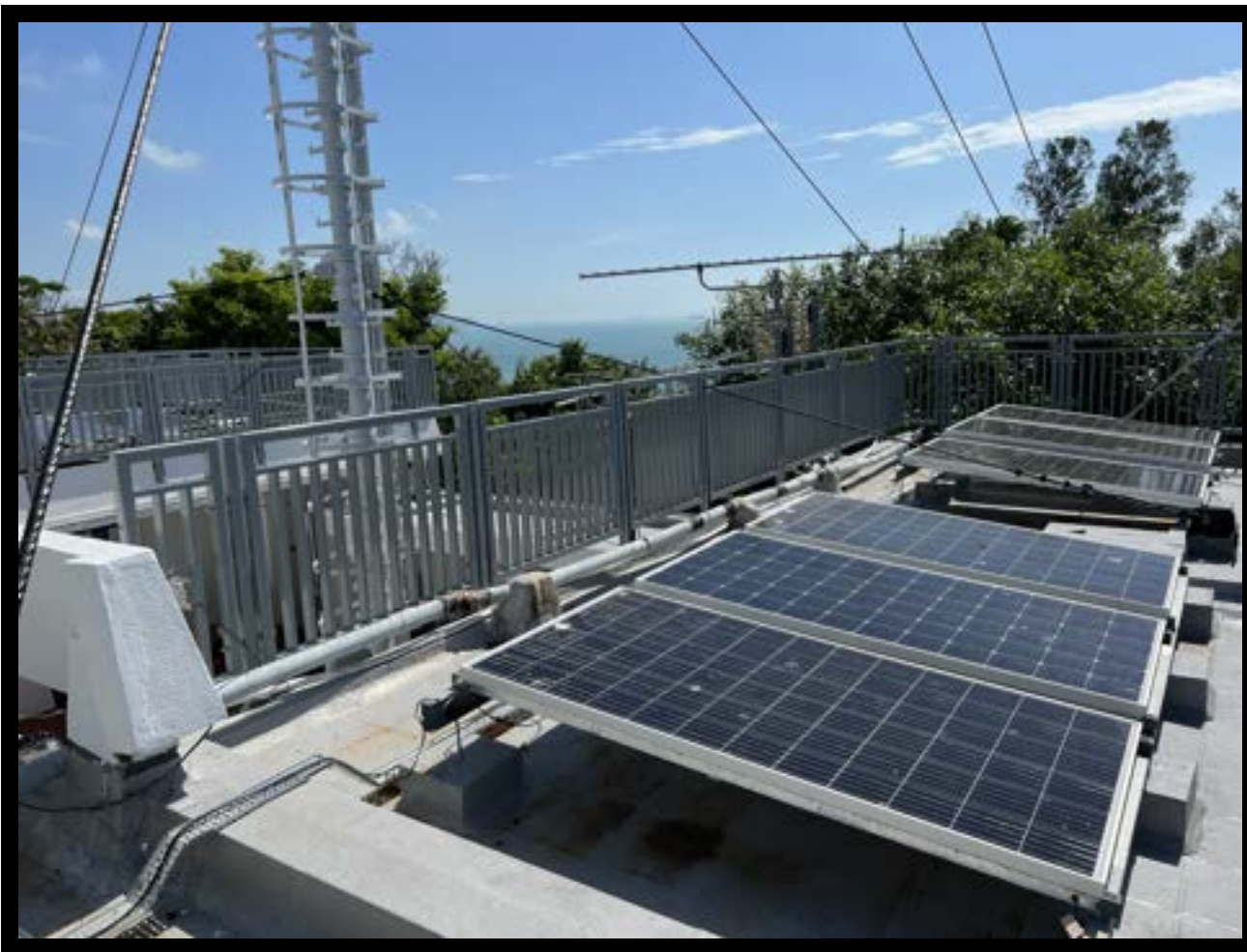
New solar power panels stated operation in Cheung Chau Meteorological Station since April 2021.
