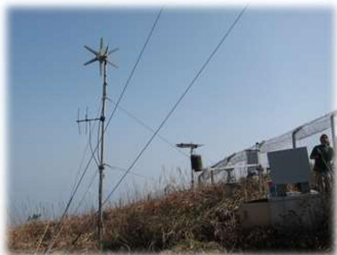
Figure 9: The automatic weather station at Nei Lak Shan using solar and wind power
