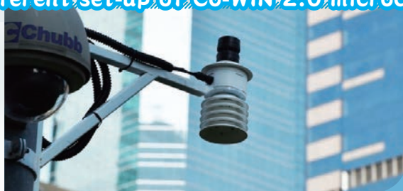
Microclimate sensors on a lamp pole
