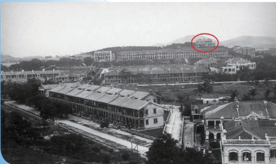
The Observatory headquarters (circled in red) in Tsim Sha Tsui, at the beginning of the 20th century (Photo courtesy of Mr Shun Chi-ming).
