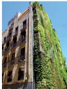
Fig 5.4 Building with vertical greening<sup>viii</sup>
