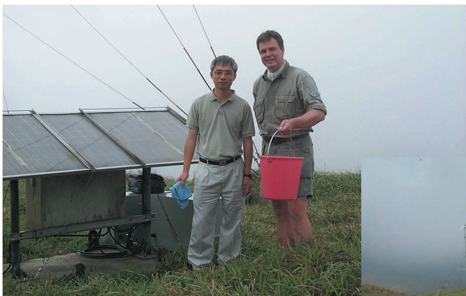
Mr Spicer and Mr Leung prepare to clean the solar panels to ensure they get adequate sunshine.
