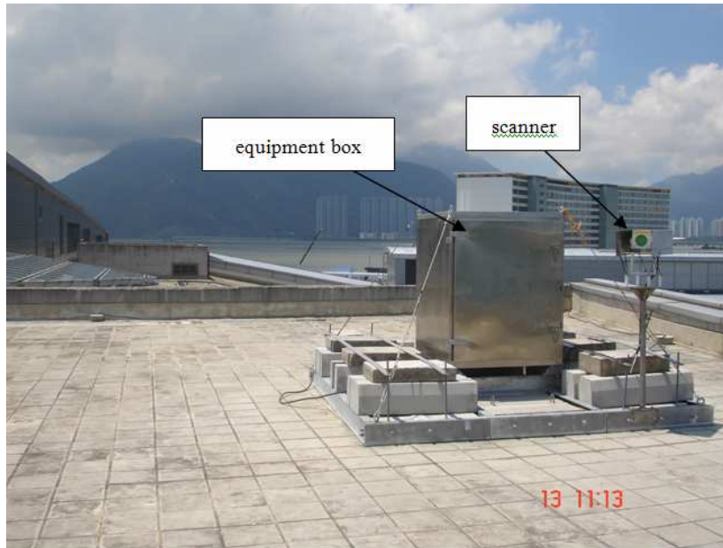
(a) The short-range LIDAR on the rooftop of an exhibition centre at the Hong Kong International Airport
