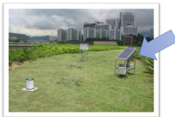
Figure 26 Automatic weather station at Lai Chi Kok Park using solar power (see arrow)
