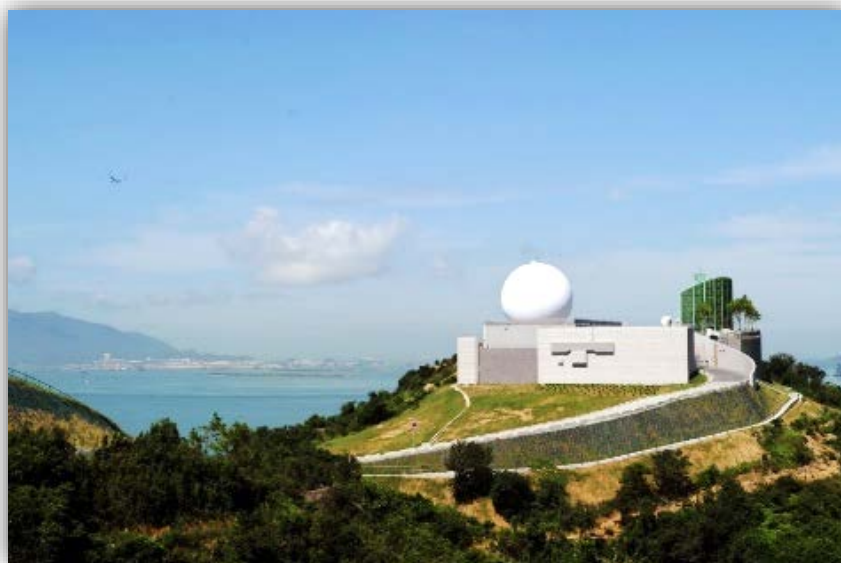
Figure 1 Brothers Point Terminal Doppler Weather Radar Station
